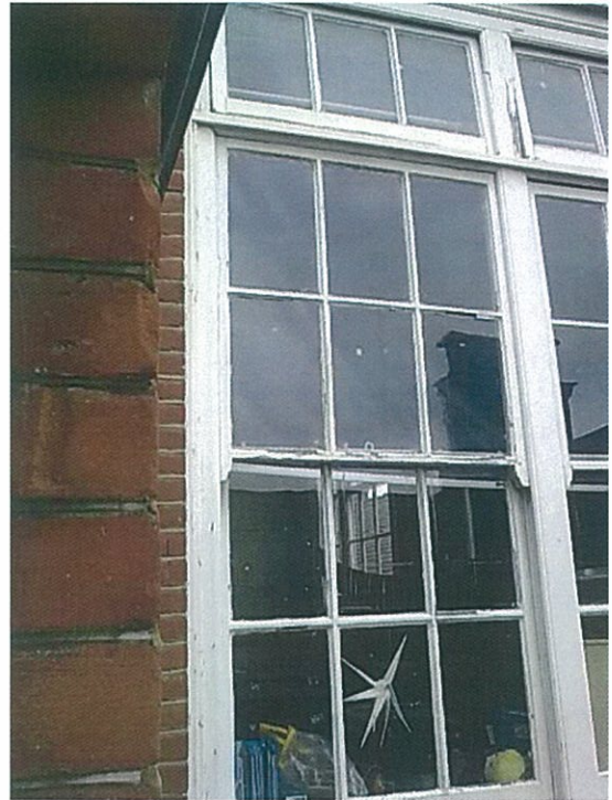
Block A – Upper Windows
