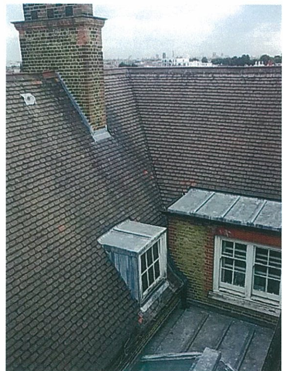
Block A – Main Roof
